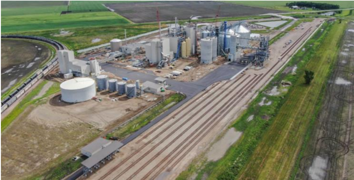
North Dakota Soybean Processors Plant, Casselton, ND Photo Credit: Jeff Beach, North Dakota Monitor
