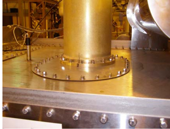
The waveguide furthest downstream on the chamber was moved toward the right.
