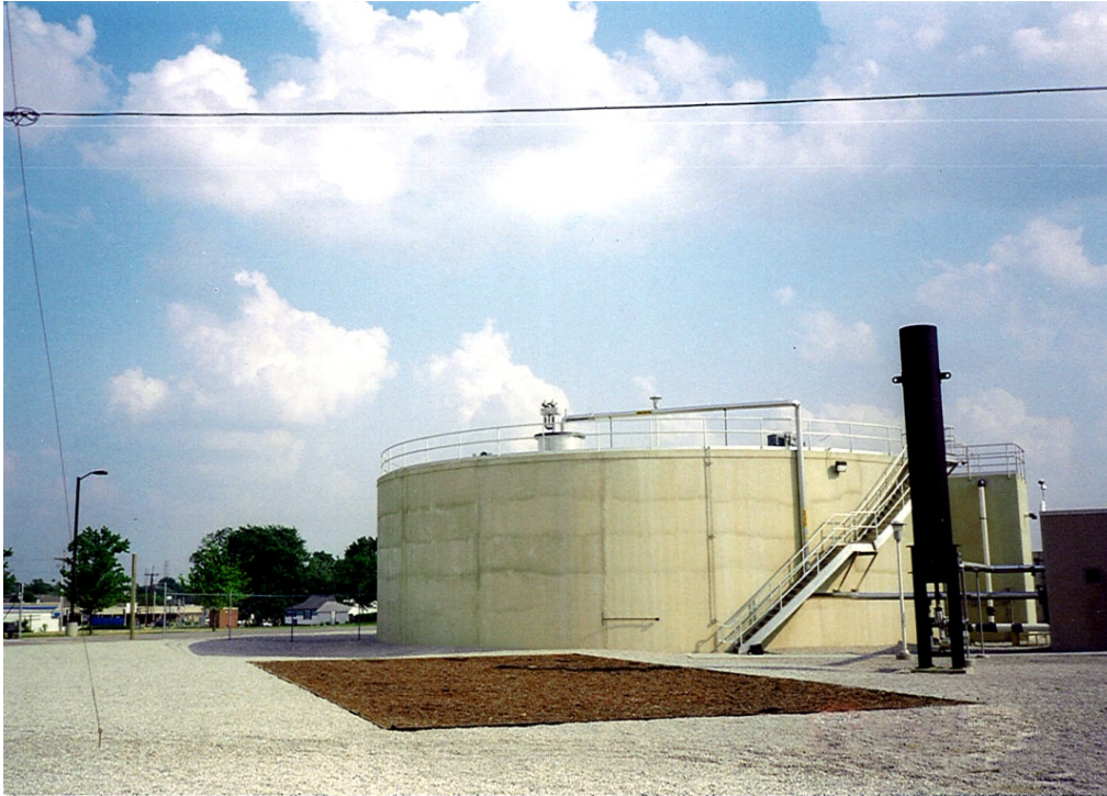
Figure 13 - General Mills Complete Mix Tank Digester. Photo courtesy of Dennis Totzke of ATI.
