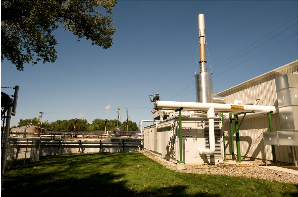
Figure 11 – Gundersen Lutheran energy generation equipment at City Brewing Company. Photo courtesy of Gundersen Lutheran.
