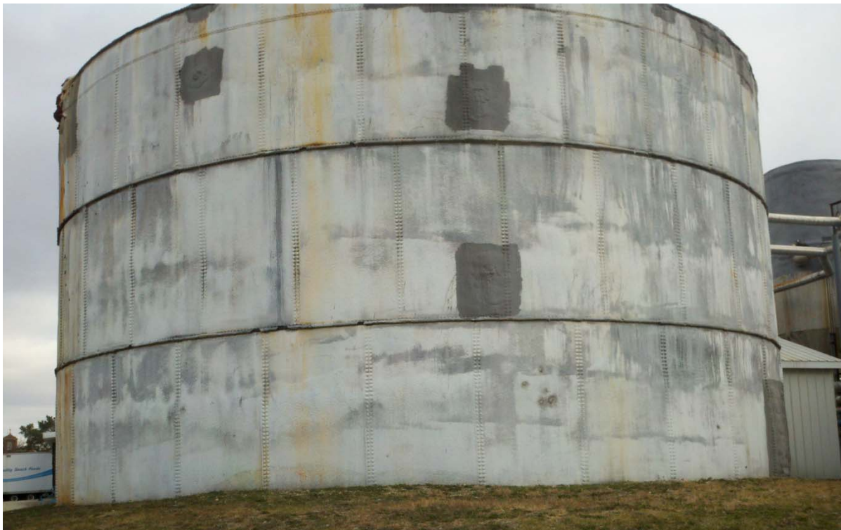
Figure 19 - Axium Foods Digester. Photo courtesy of Axium Foods.
