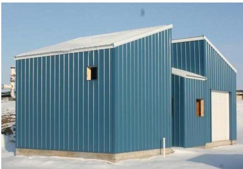
Figure 28 - Building with gas conditioning and compression equipment. Photo courtesy of SunOpta.
