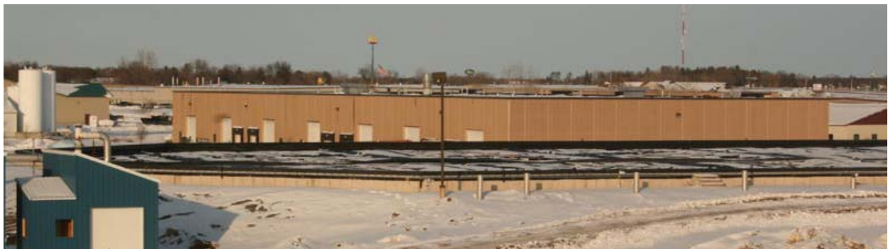
Figure 27 - SunOpta UASB digester. Photo courtesy of SunOpta
