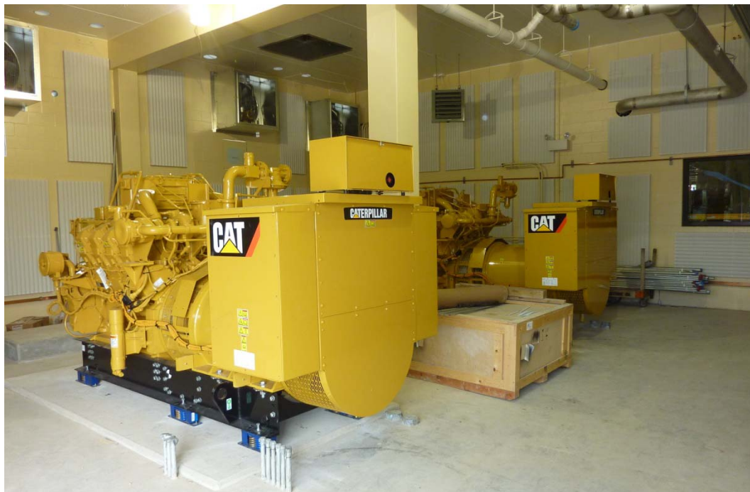
Figure 10 - Engine generator sets at Beaver Dam. Photo courtesy of Wayne Karlovich, Applied Technologies, Inc.
