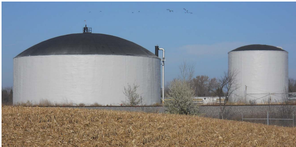
Figure 15 - JBS-Green Bay anaerobic contact process digester and equalization tank. Photo courtesy of JBS Green Bay.
