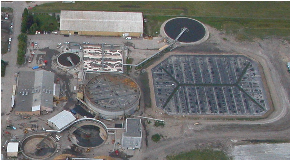
Figure 6 - American Crystal Sugar Company East Grand Forks Facility. Photo courtesy of American Crystal Sugar Company.
