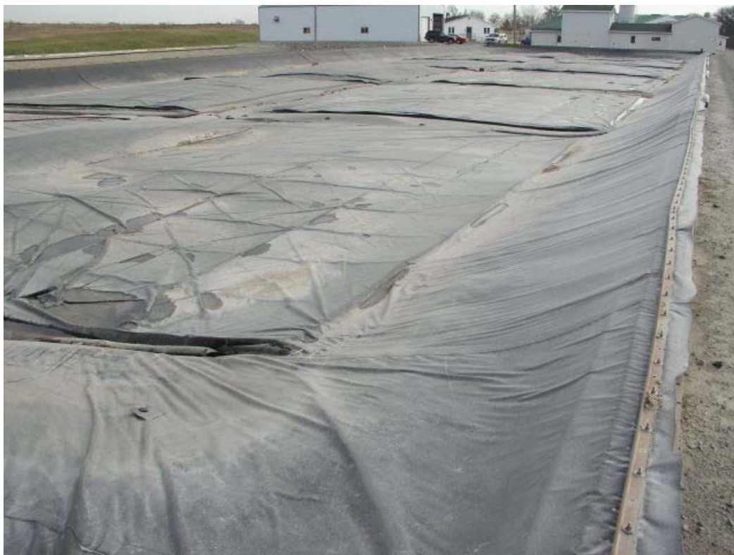
Figure 24 - Mixed, heated covered lagoon digester. Photo courtesy of Saputo Cheese USA, Inc..
