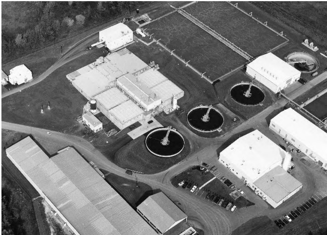
Figure 7 - Anheuser Busch Baldwinsville Facility. Photo courtesy of Anheuser Busch.
