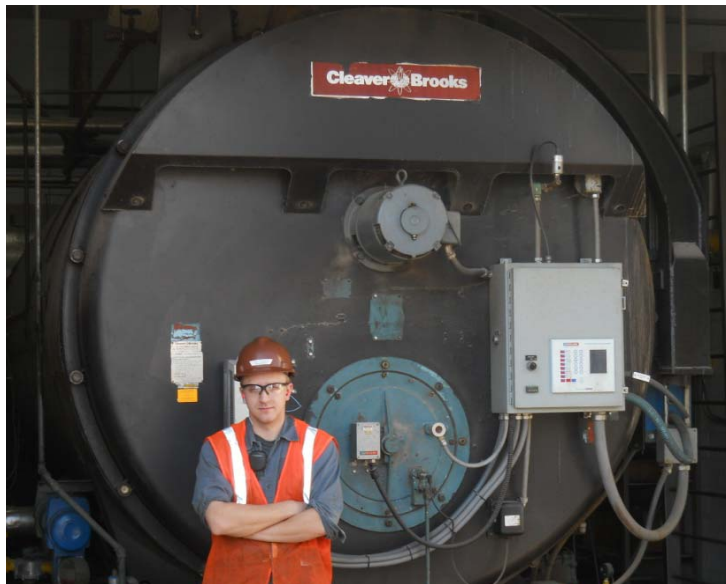
Figure 16 - JBS Green Bay dedicated biogas boiler and operator Paul Wandrey. Photo courtesy of JBS Green Bay.
