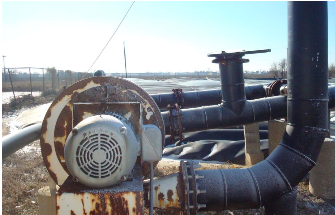
Figure 22 - Monmouth North Pretreatment Plant Gas Handling Equipment, courtesy of Cliff Haefke, US DOE Midwest RAC.
