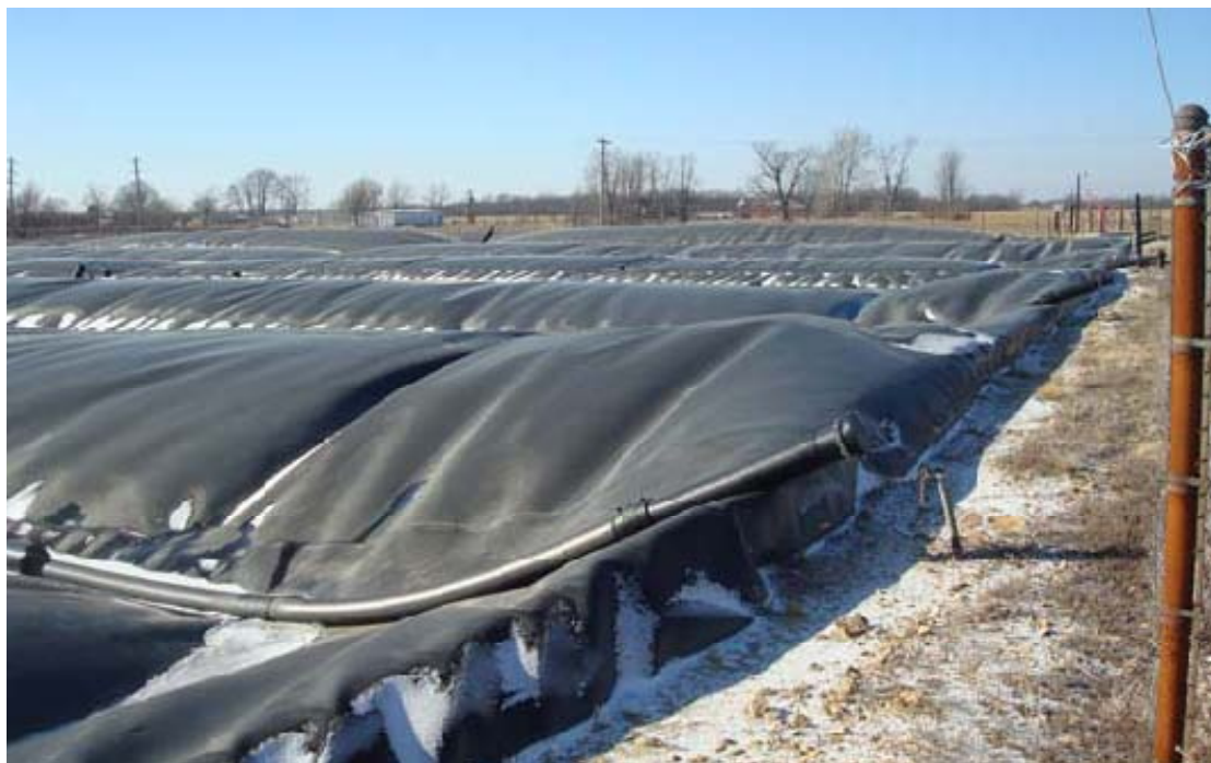
Figure 21 - Monmouth North Pretreatment Plant Covered Lagoon. Photo courtesy of Cliff Haefke, US DOE Midwest RAC.
