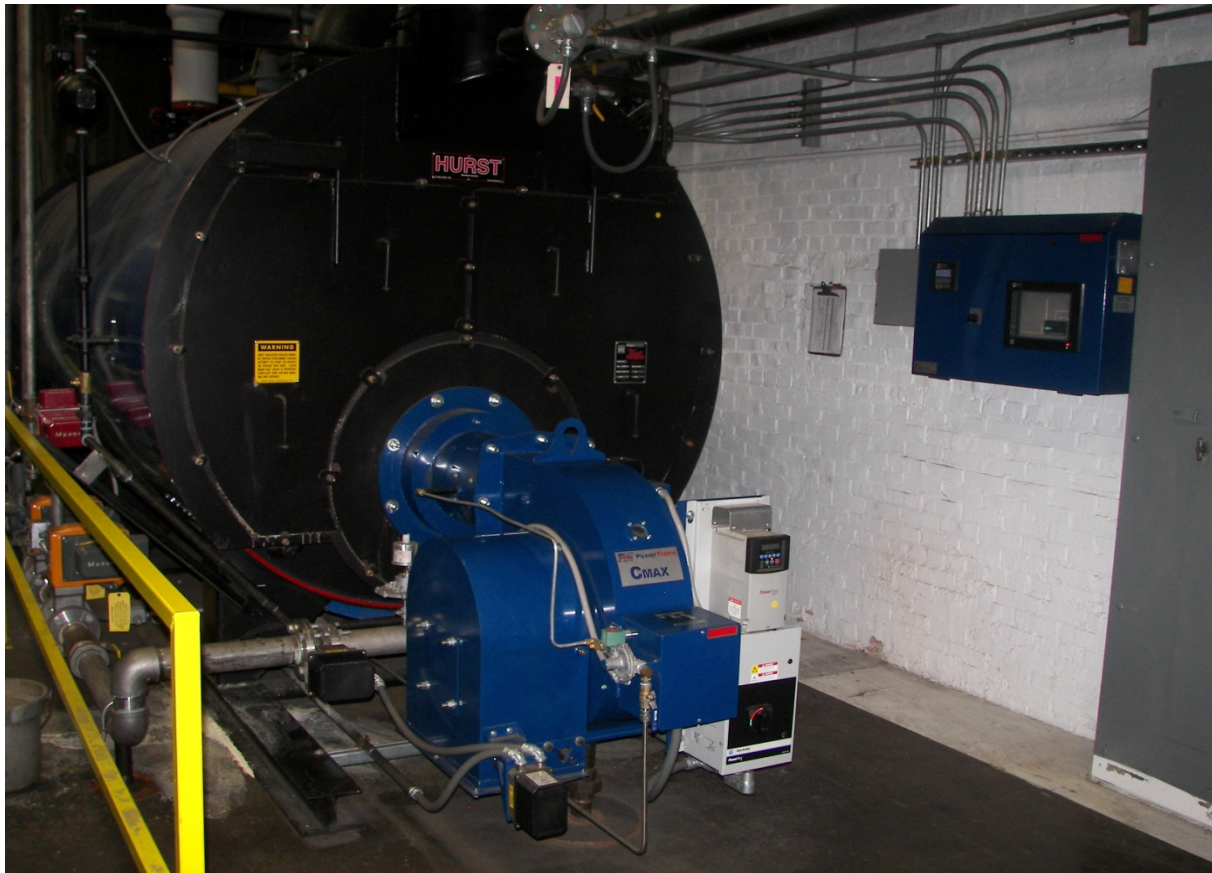
Figure 26 - Biogas hot water boiler. Photo courtesy of Seneca Foods.
