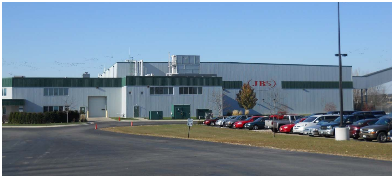
Figure 14 - JBS Green Bay product distribution facility. Photo courtesy of JBS Green Bay.
