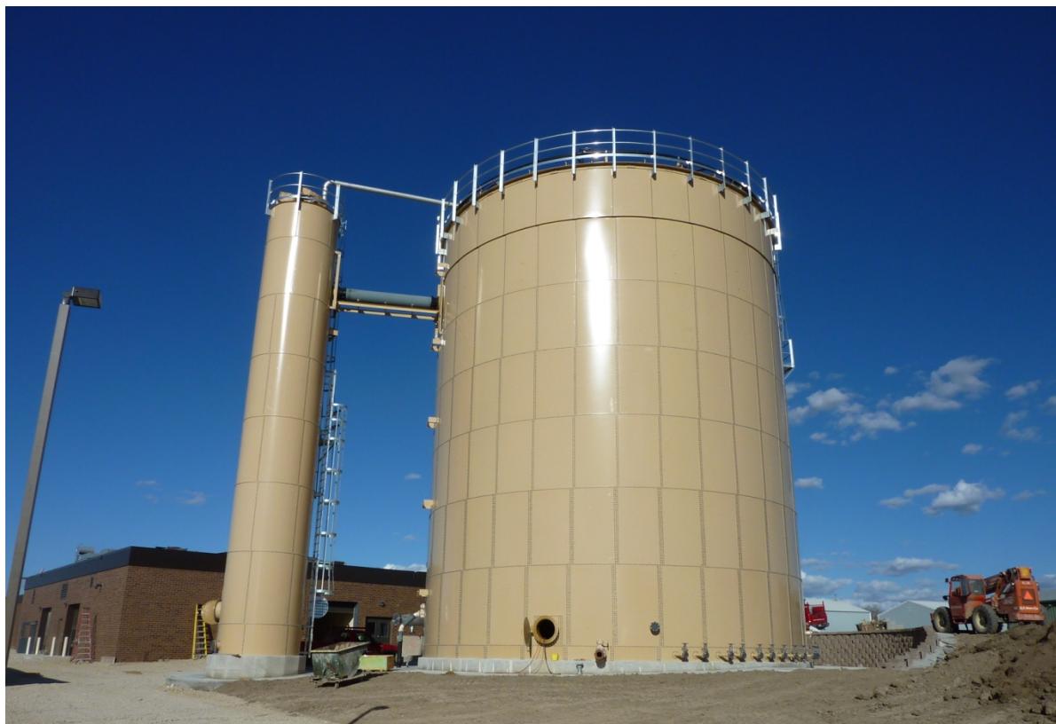
Figure 9 - Beaver Dam UASB Digester during construction. Photo courtesy of Dennis Totzke, Applied Technologies, Inc.
