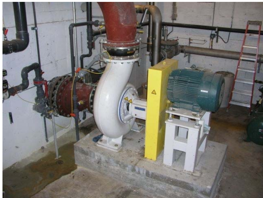
Figure 23 - Mixing pump for digester. Photo courtesy of Saputo Cheese USA, Inc.
