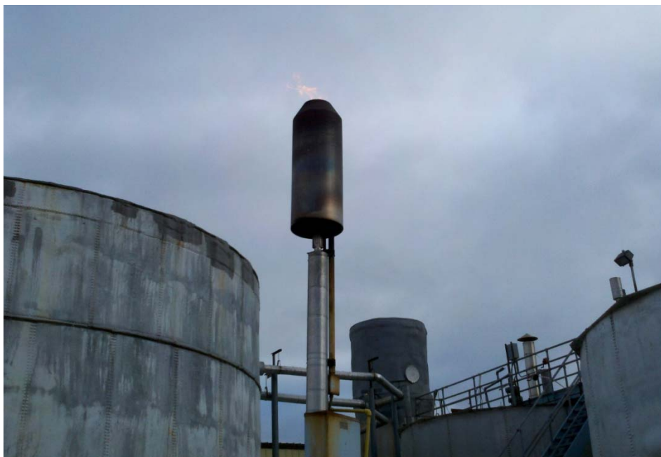
Figure 20 - Biogas flare. Photo courtesy of Axium Foods.
