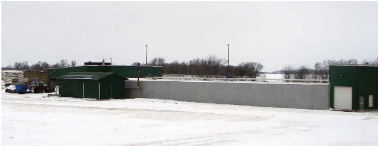
Figure 25 - Seneca Foods Digester. Photo courtesy of Seneca Foods.
