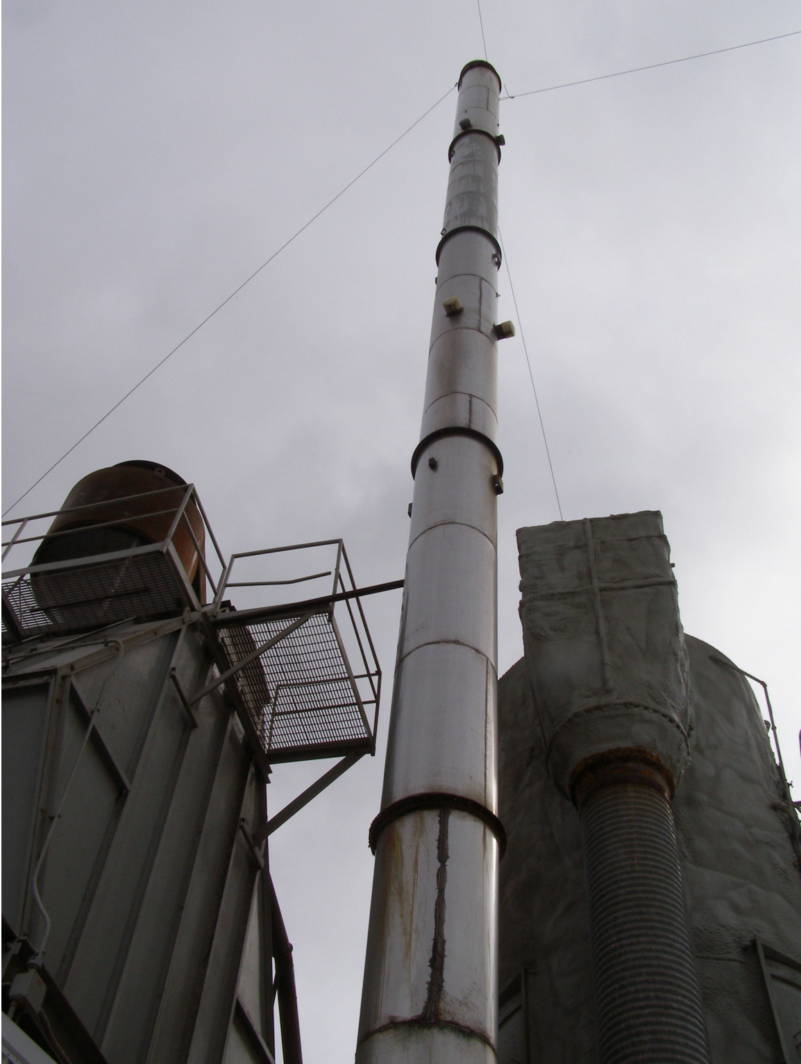
Picture 7: Van der Geest Dairy: a baghouse with 376 polyester bags is needed to control particulate levels well enough to meet DNR requirements for the dryer's emissions.
