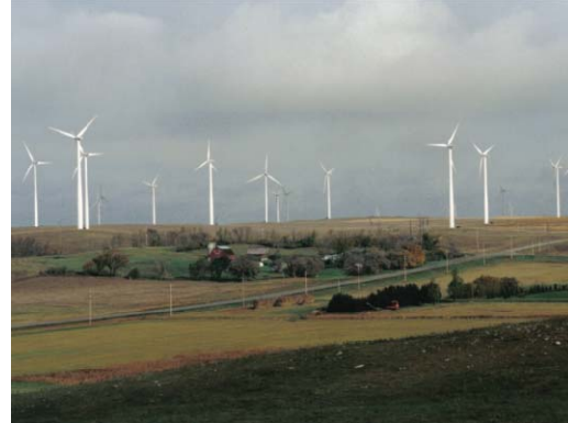
Large wind farm requiring high voltage transmission for interconnection and delivery of power. Southwest Minnesota
