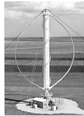
U.S. D.O.E.'s 500-kW variable speed vertical axis Darrieus wind turbine
