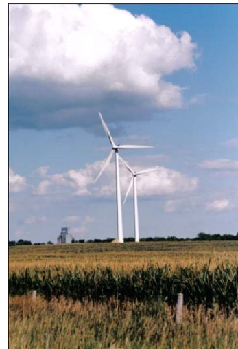
Small cluster of turbines Connected to distribution level voltage. Southwest Minnesota
