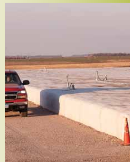
Riverview, a 30,000-cow dairy, installed three anaerobic digesters to produce methane from manure. The company has started marketing leftover digester solids as a soil amendment for gardens.
