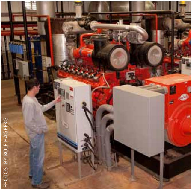
A generator at Riverview dairy produces 3.6 megawatts of electricity from methane pumped in from anaerobic digesters.
