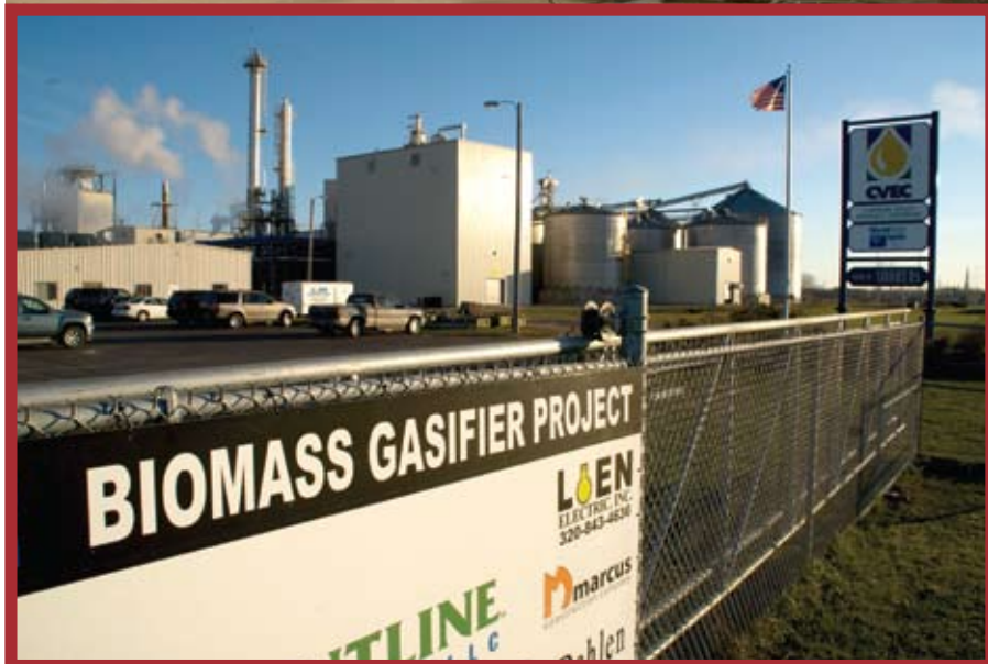
A biomass gasifier, the large cylinder rising in the center of the photo above, will replace about 20 percent of the Chippewa Valley Ethanol Company's energy consumption when it goes online in early 2008. Eventually gasification will supply all of the plant's energy needs.
