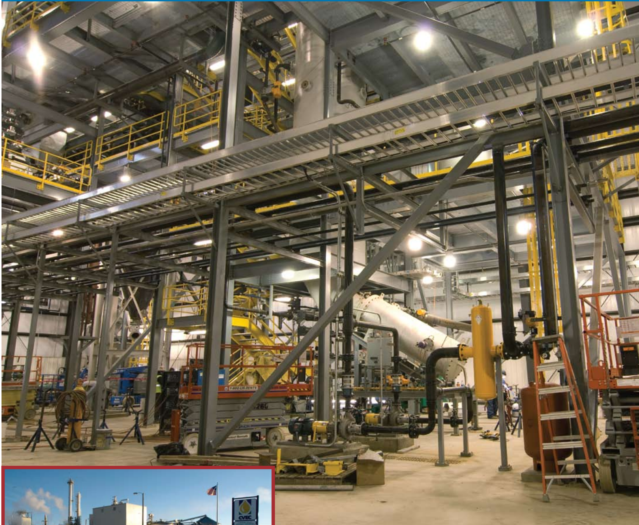
A biomass gasifier, the large cylinder rising in the center of the photo above, will replace about 20 percent of the Chippewa Valley Ethanol Company's energy consumption when it goes online in early 2008. Eventually gasification will supply all of the plant's energy needs.
