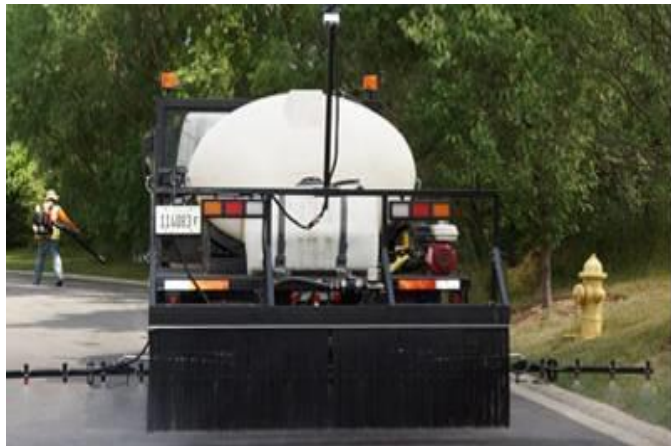
Pavement Seal Coating
