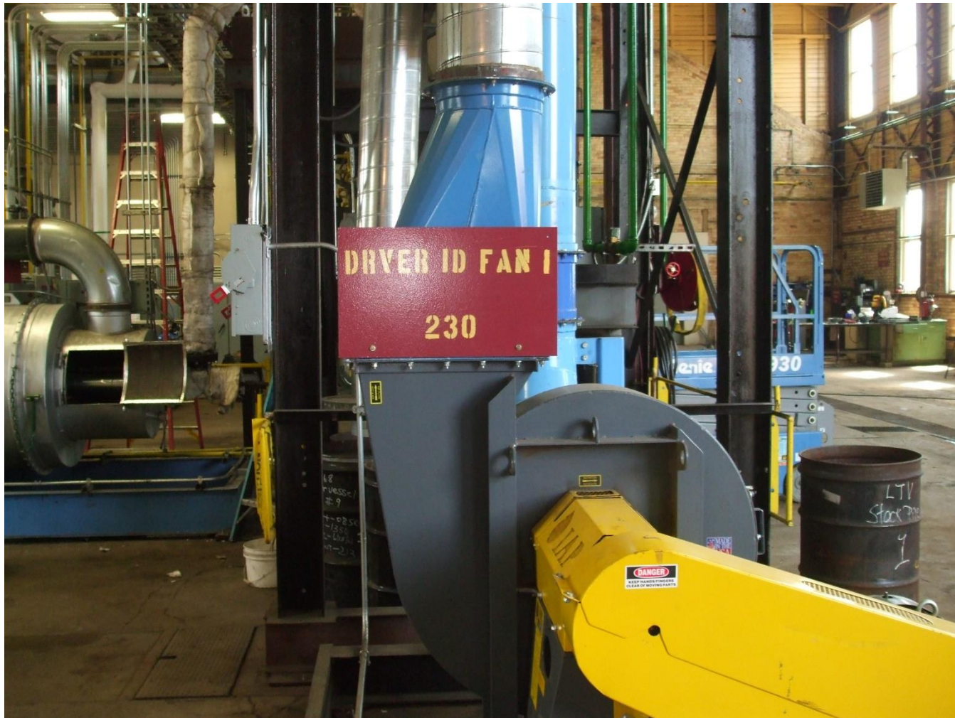
ID Fan Used to Drive Pneumatic Transport from Dryer to Cyclone
