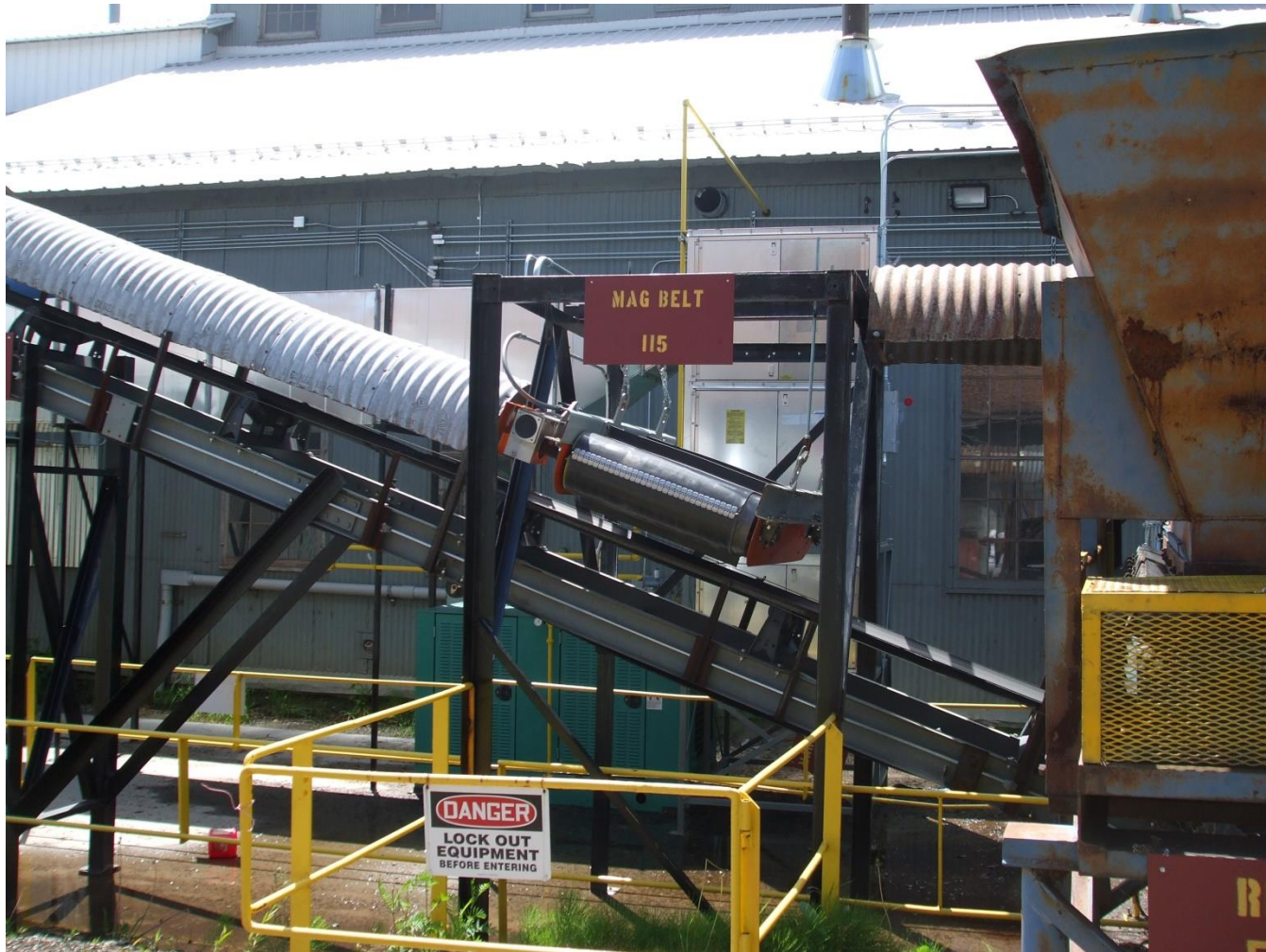
Conveyor to Shaker Screen and Tramp Metal Magnet
