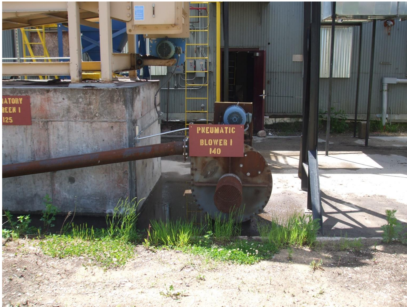
Pneumatic blower for transport of sized materials
