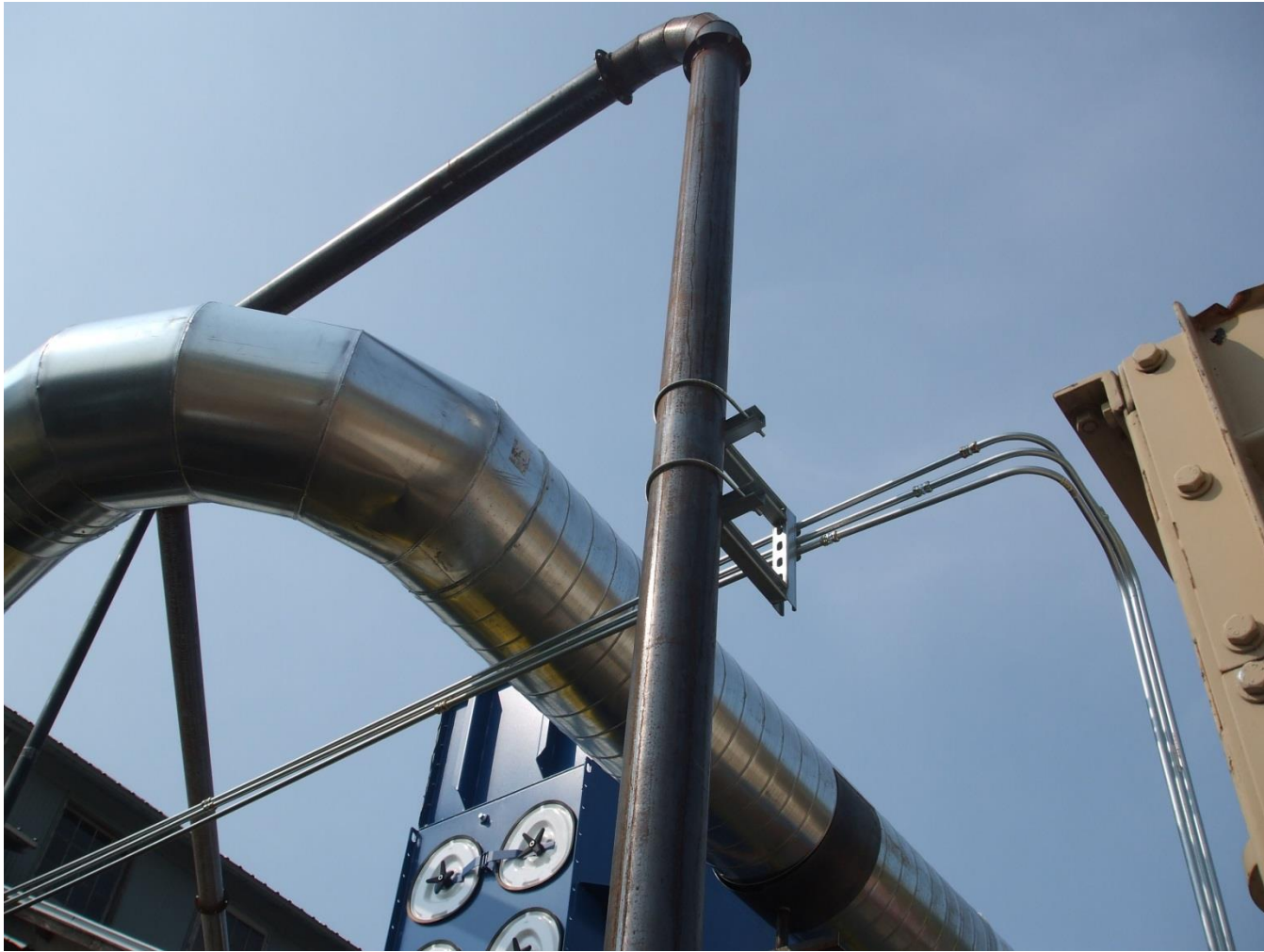
Pneumatic transfer piping and air movement ducting
