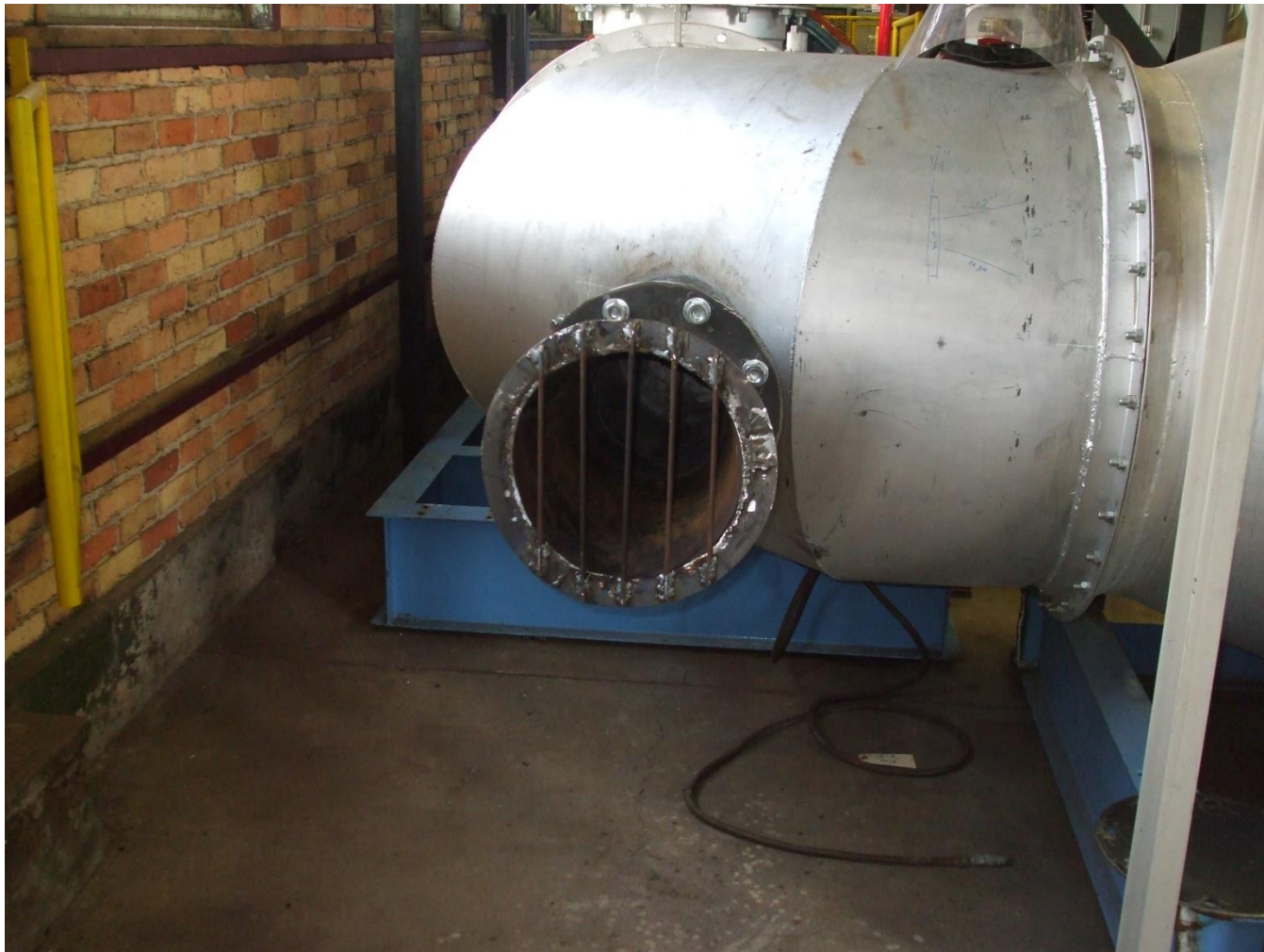
Port for Air Modulation at Combustion Chamber Exit
