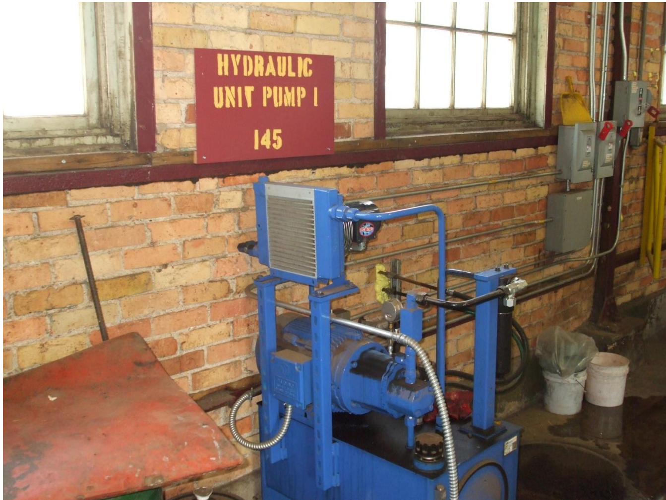
Hydraulic System Used for Moving Floor Trailers
