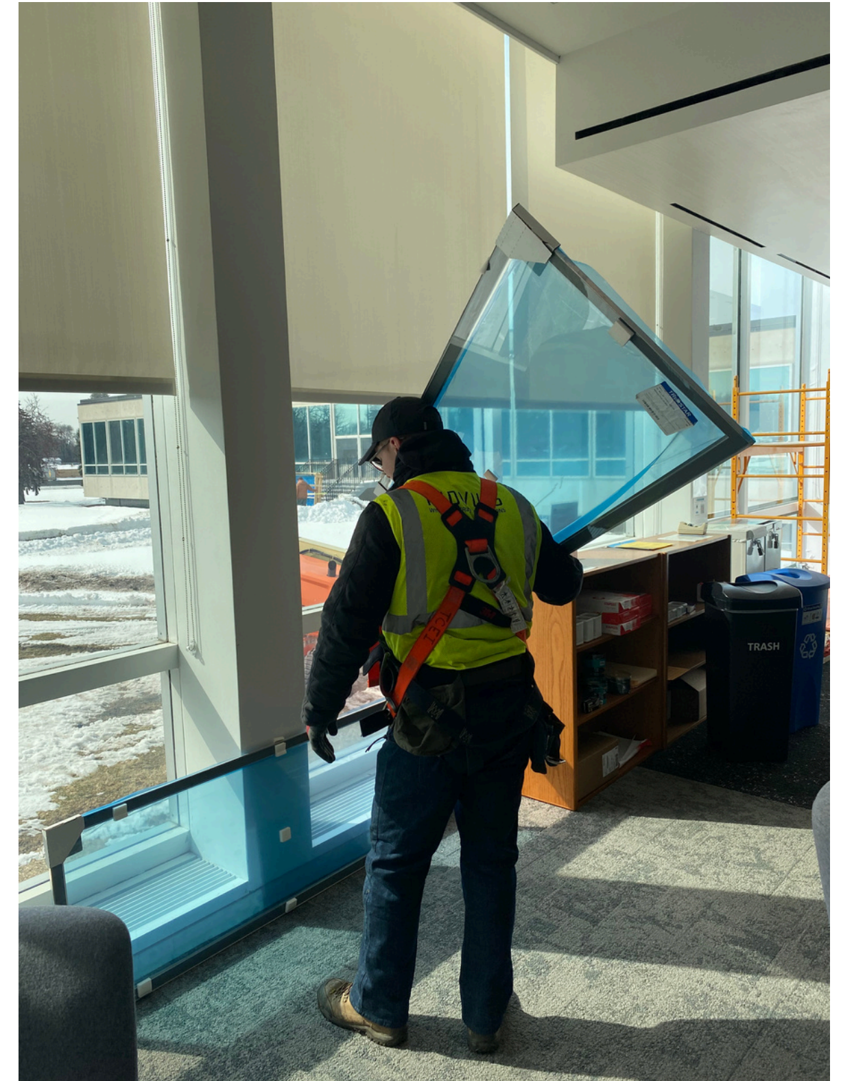
INOVUES window installation on the 3M campus in 2023
